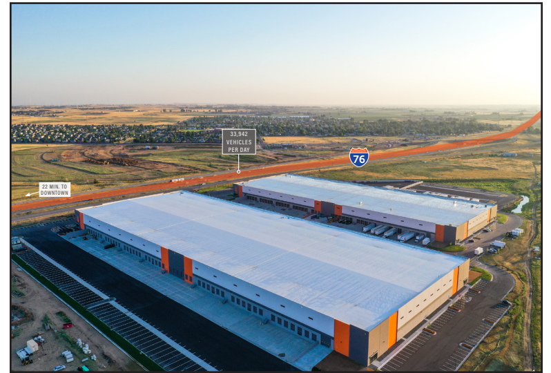
Principal Real Estate Investors purchased Buildings 4 and 5 at 76 Commerce Center.
